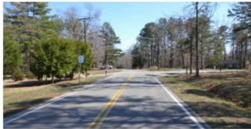
Existing Conditions - Looking East From Old Hundred Road
